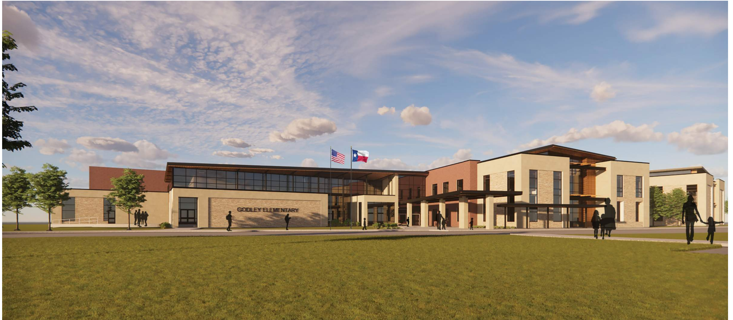
OVERALL EXTERIOR VIEW
